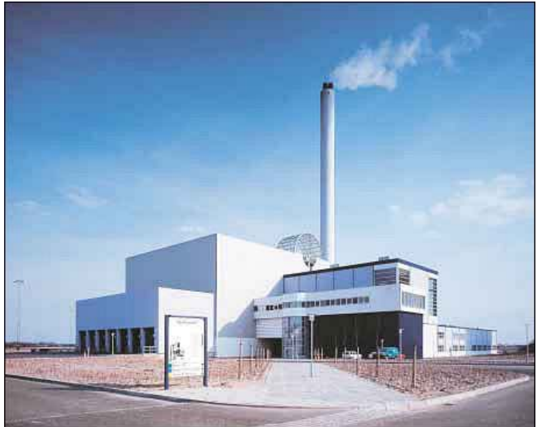
The Danish waste incineration plant Måbjergværket is to be modernised to meet the new EU directives concerning hazardous emissions. The energy company Elsam will also be upgrading four other similar plants in Denmark. Photo: Elsam.
