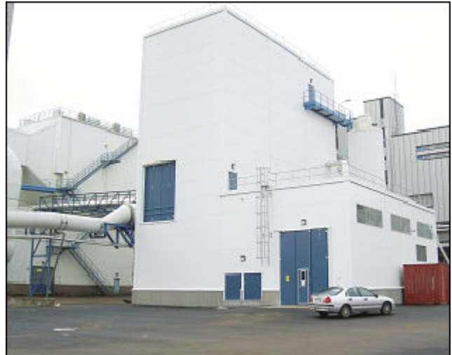
The expansion of Hedenverket has meant the erection of a completely new building.
