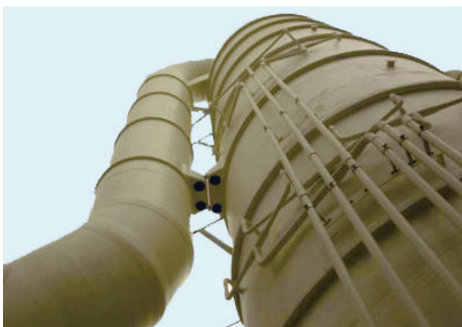
Multifunctional condensing scrubber at SYSAB in Malmö, Sweden, with ADIOX® for memory effect prevention.
