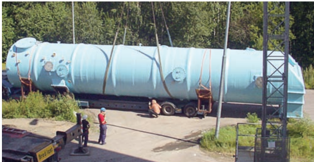
Transporting a scrubber incorporating ADIOX® for memory effect prevention to a waste incinerator in Karlstad, Sweden.
