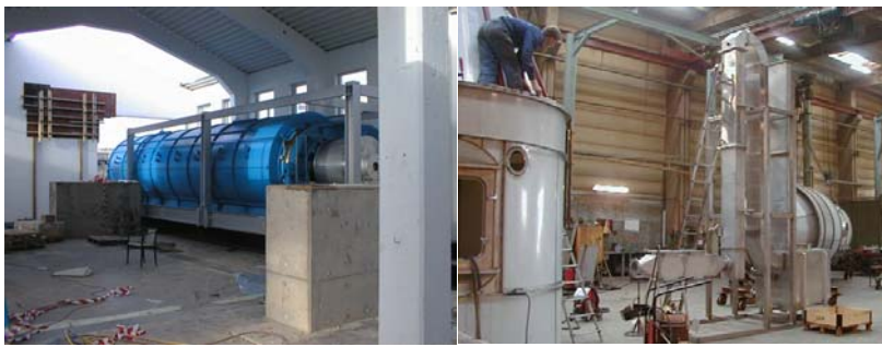
Rotary kiln during erection
