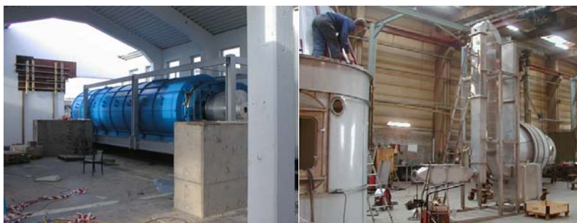
Roterugn under montage
