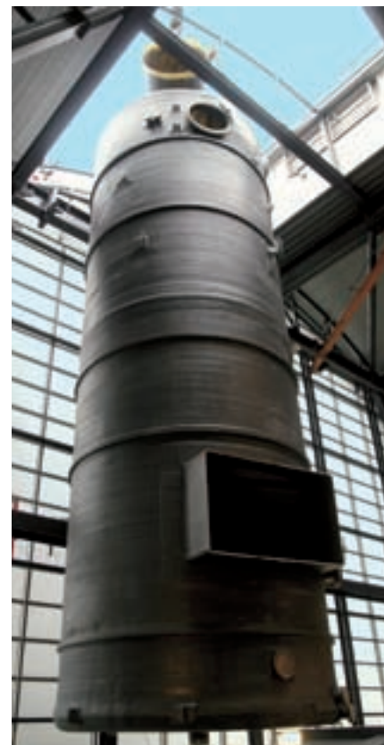
The condensing scrubber is lifted into place at Sønderborg KVV in August.
