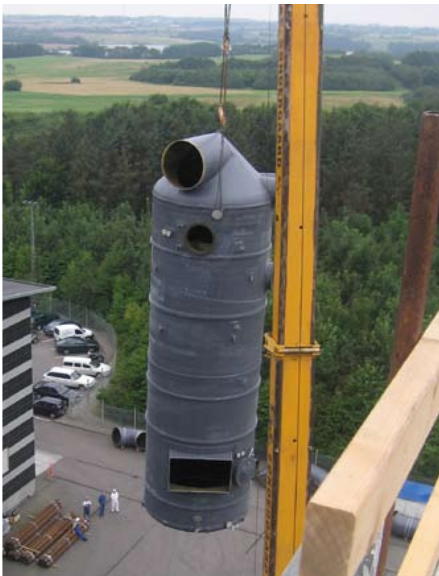
The condensing scrubber is lifted into place at Sønderborg KVV in August.
